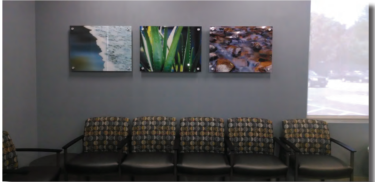
Acrylic Pieces Installed
